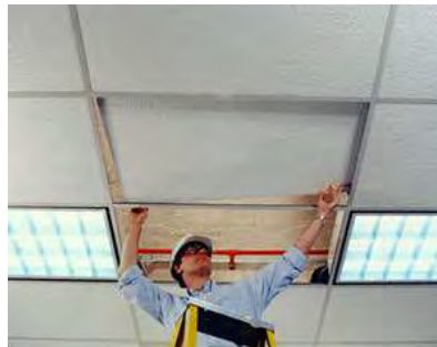
FIG. 14 - Tilt the FRP ceiling panels slightly and drop them into position.
