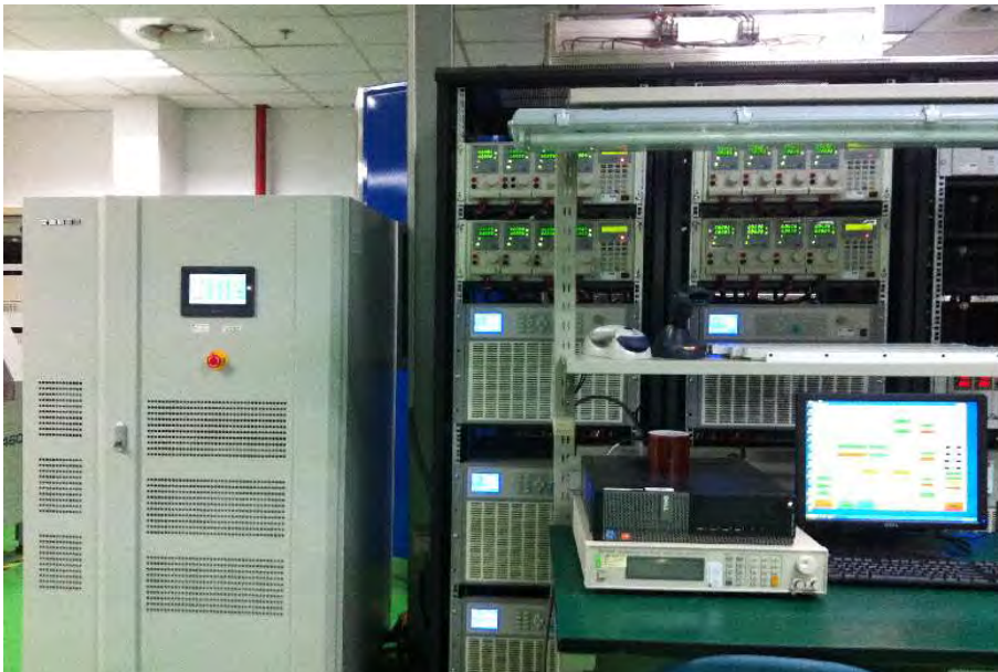
Server Power Supply Test
