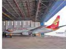
Aircraft Maintenance Plant
