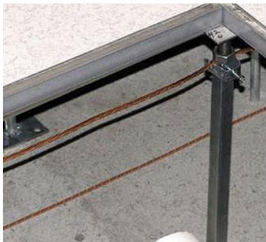
Figure 4. Ground wire in subfloor
