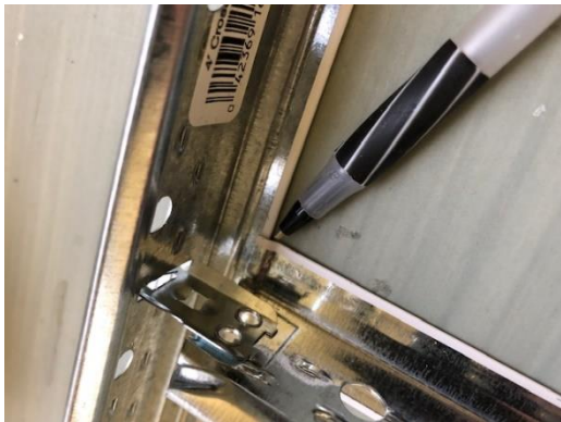
Cross Tee to Main Beam Intersection
