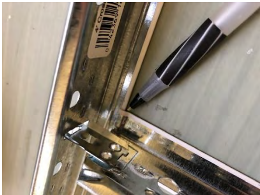
Cross Tee to Main Beam Intersection
