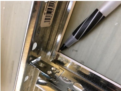
Cross Tee to Main Beam Intersection
