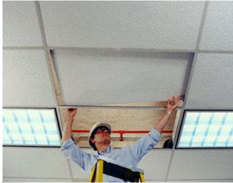
FIG. 14 - Tilt the ceiling panels slightly and drop them into position.
