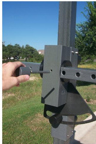
2. Remove polarization locking pin.
