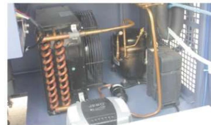
Chamber of imported compressor refrigeration system consisting of cascade refrigeration system
