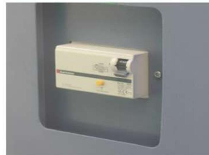
Leakage protection switch for leakage fault occurs in the device and the other shock protection
