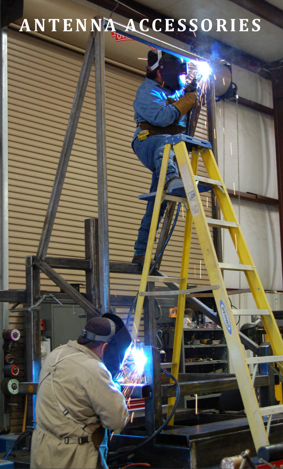
Welding the HO-2450-15 Horn Trailer Pedestal
