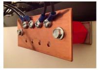
Figure 5. Ground bar Source: www.copper.org
