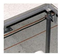
Figure 4. Ground wire in subfloor
