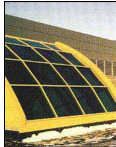
The Registry Building at the FAA Mike Monroney Aeronautical Centre, Oklahoma City, USA. Architect: Frankfurt Short Bruza. Datastop installed to protect computerized records from nearby radar system.
