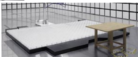
Installation of wave absorber is completed.
