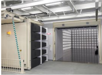
Sliding is completed barrier-free open status
