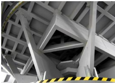
View of the lower structure from the pit. This entire structure rotates in the new system.
