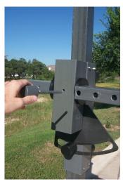
2. Remove polarization locking pin.
