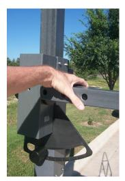
With pin removed, grasp mounting arm.
