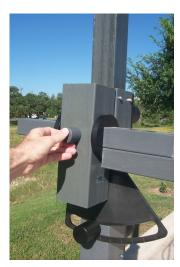
5. Replace polarization locking pin.
