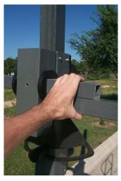
4. Manually rotate mounting arm 90 degrees counterclockwise.
